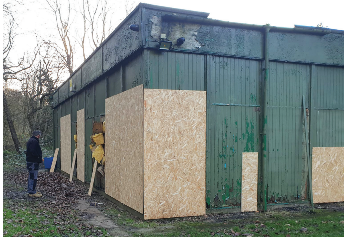
Work in progress to remove old panels
